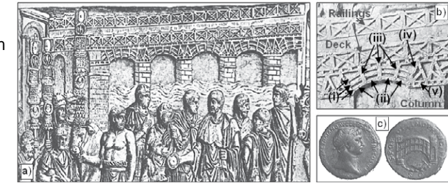
A carving from Trajan's Column in Rome (at left and upper right) and a contemporary Roman coin provided clues to the bridge's form. (Images courtesy of Branko Glišić)
